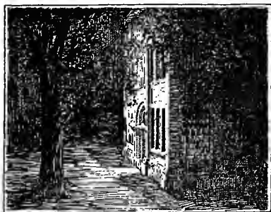
ENTRANCE, RAND HALL, NIGHT
